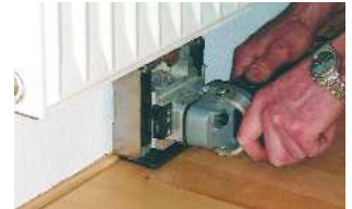
Cutting expansion joints
