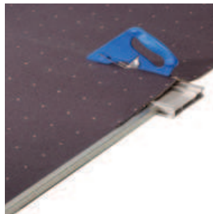
Cutting on the floor with USF. A squaring guide and hand cutter are also pictured.
