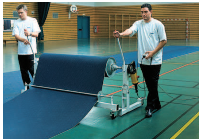
On-Rolling with Transport and Unroll Trolley with the electric winding motor
